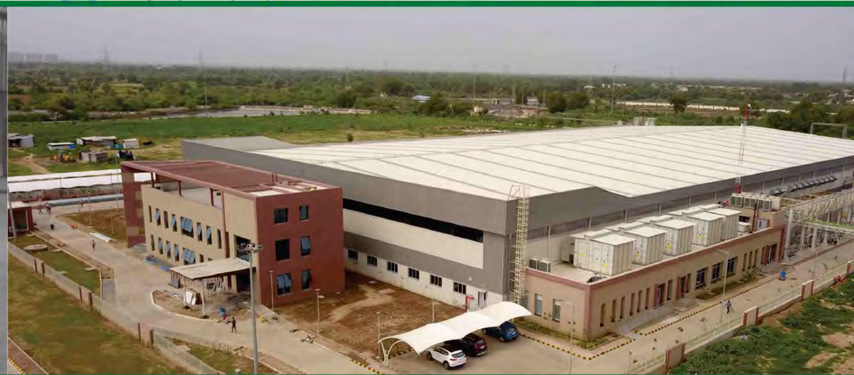
Aerial view of IFFCO's Nano Urea plant in Gujarat
